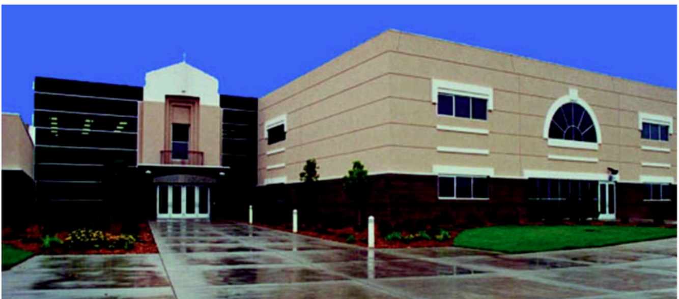
Lucile Erwin Middle School features an ASHRAE Technology Award-winning hybrid chilled water/ice thermal storage plant
